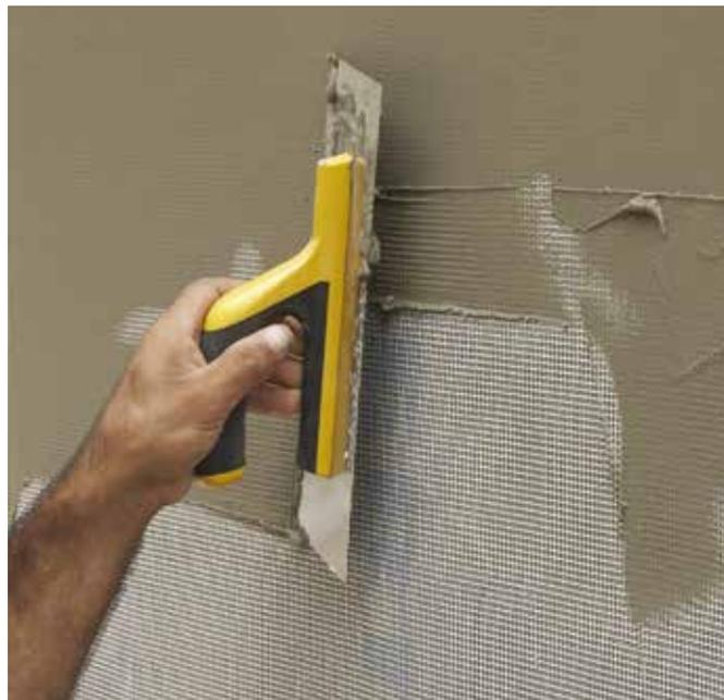
side of the joint) Reinforcement with flexible tape or alkali resistant reinforcement mesh should be performed in order to prevent any cracks if the panels move. Reinforcement is embedded in the plaster, when the plaster is still wet, as recommended by the reinforcement manufacturer.
